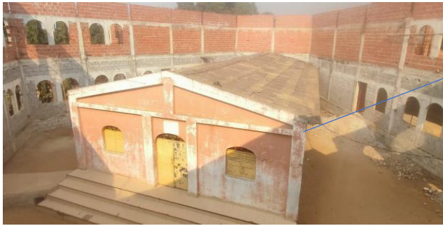
part under construction
